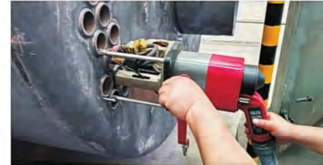
△自动管板焊 Automatic Tube-To-Sheet Welding
