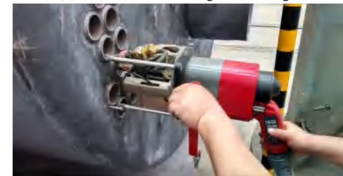
△自动管板焊 Automatic Tube-To-Sheet Welding
