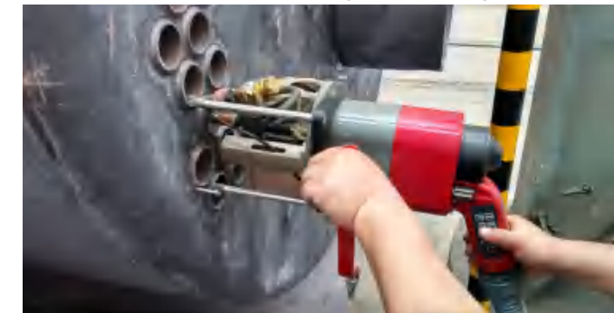
△自动管板焊 Automatic Tube-To-Sheet Welding
