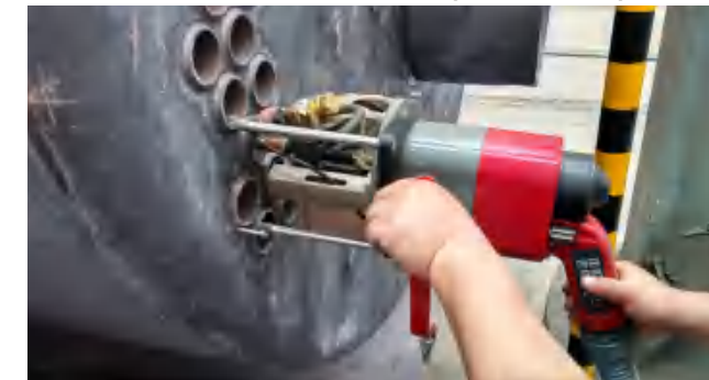
△自动管板焊 Automatic Tube-To-Sheet Welding
