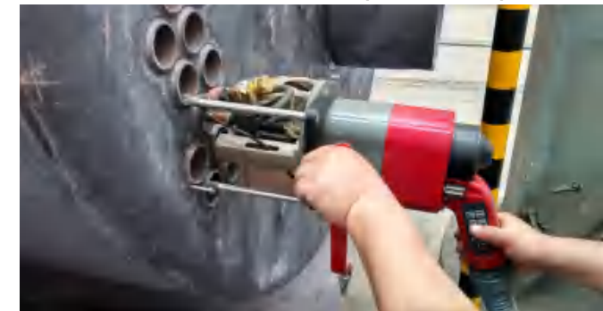
△自动管板焊 Automatic Tube-To-Sheet Welding
