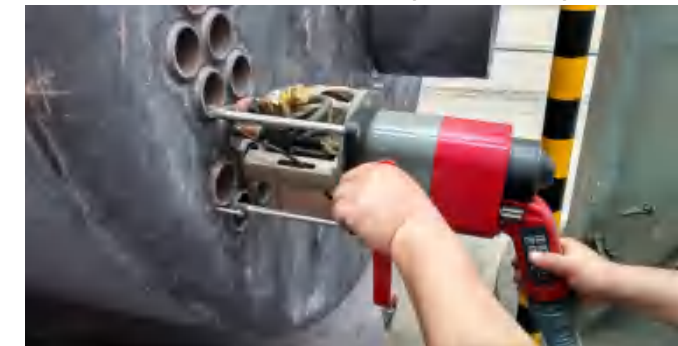
△自动管板焊 Automatic Tube-To-Sheet Welding
